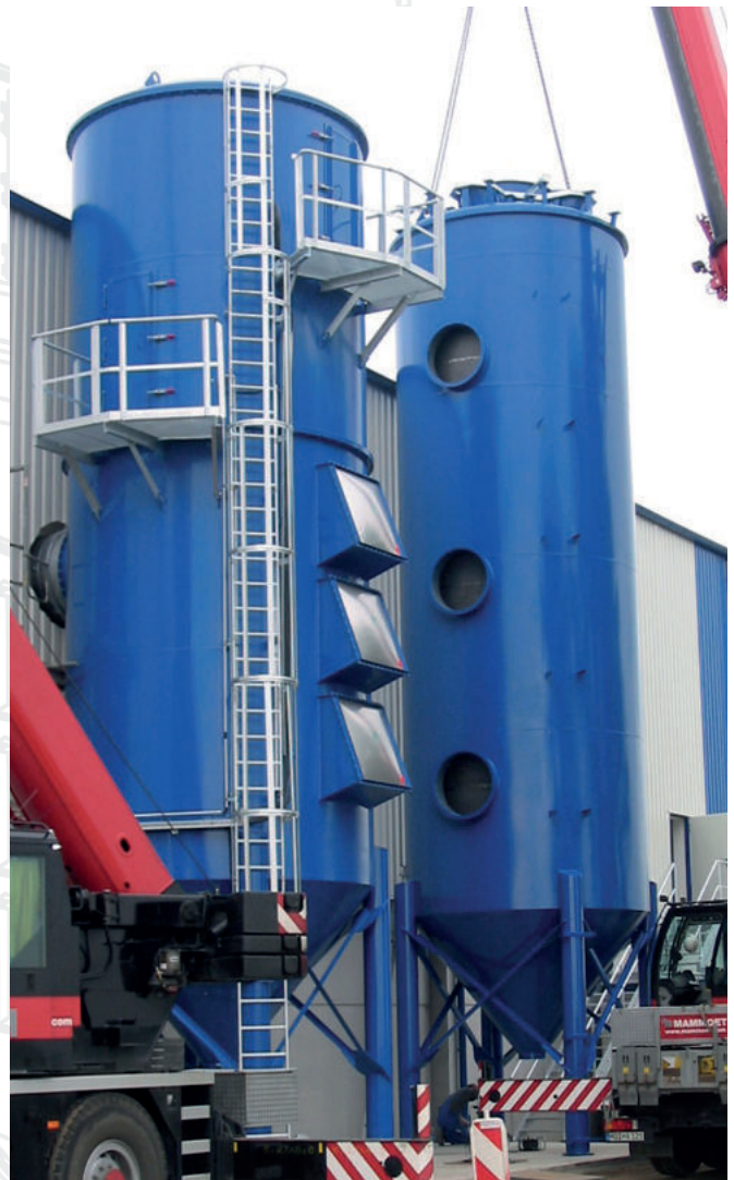
Transport/Assembly of a bag filter and activated carbon filter
